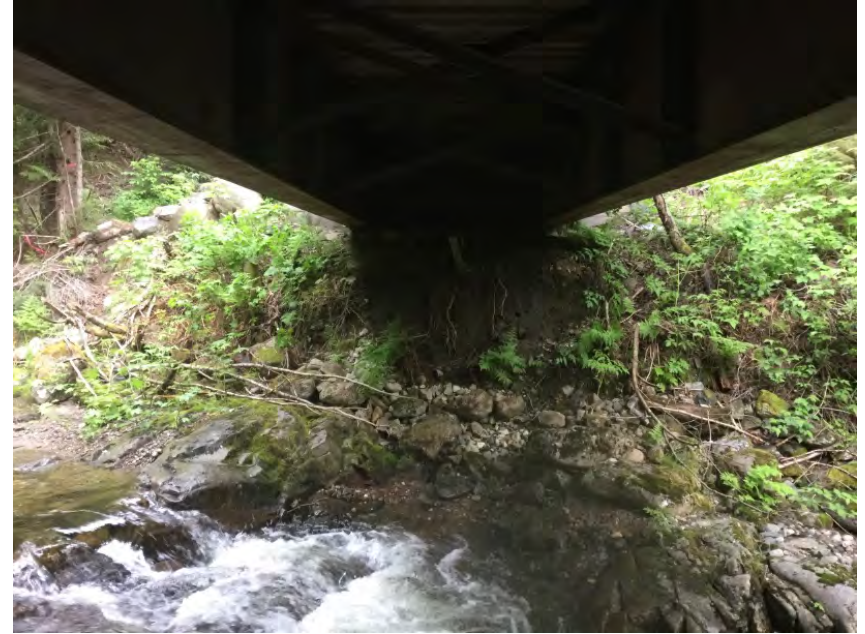
Left Bank Abutment when facing downstream
