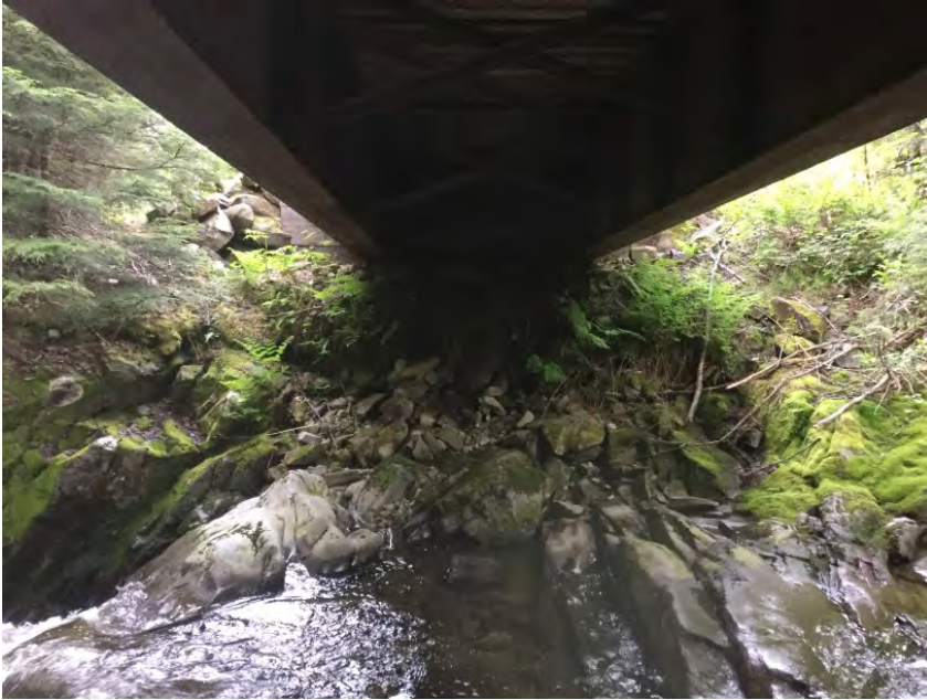
Right Bank Abutment when facing downstream
